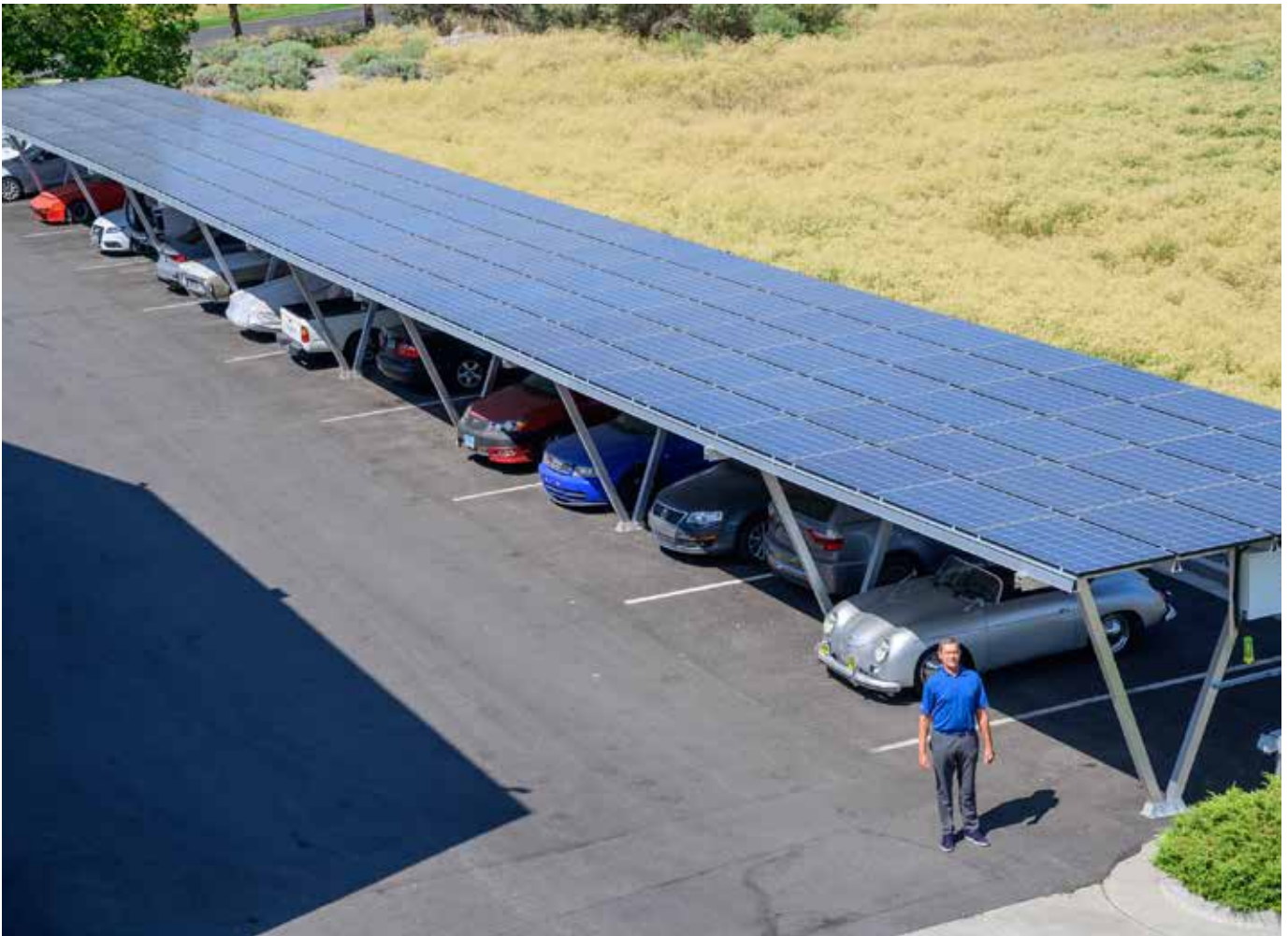
270 solar panels line the carport at de Jong's headquarters. The building is entirely off-grid, with solar power used as its primary energy
