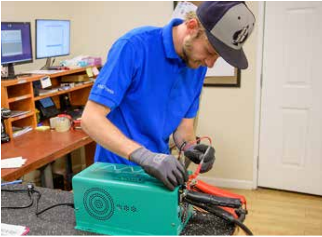
Jepsen examines an inverter sent to Aims Power for warranty repair.
